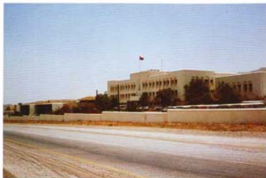
Muscat Water Supply Improvements
