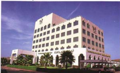
British Bank of the Middle East H.Q. Ruwi
